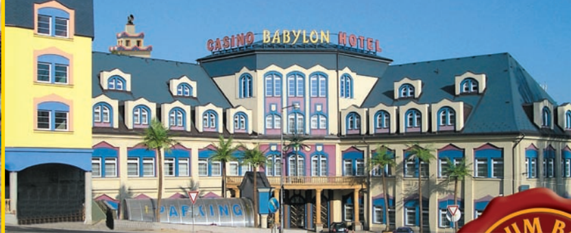
ALL UNDER ONE ROOF
